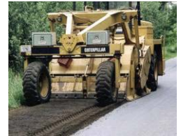
Recycled Asphalt Road Dust Control Road Reclamation Milling Stabilization
