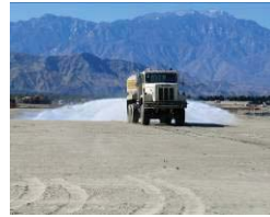
Land Development Fugitive Dust Control Erosion Control Silt Loading Control
